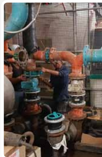
Remove old valves and replace pump valves with the new ones to avoid pipeline breakage and water leakage.
